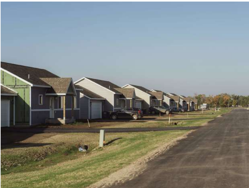
New housing being built amid a population increase related to the new data center.
